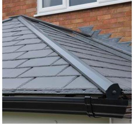
Ultrarroof offers a magnificent vaulted plastered ceiling on the inside enhancing the feeling of space within your current conservatory. **Thermally efficient with a U-value of 0.16**, Ultrarroof offers you the warmth and brightness you require, with beautiful and authentic looking lightweight tiles externally, with the option for full height glazing to flood your home with light and create a stunning feature.
